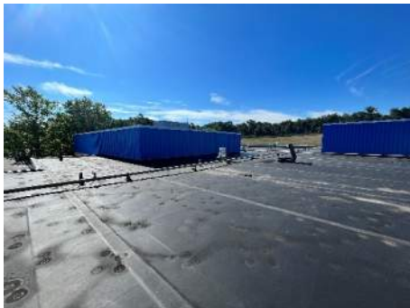
Single-ply roof membrane
