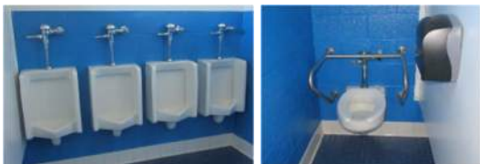
Existing Gang Toilet Plumbing Fixtures
