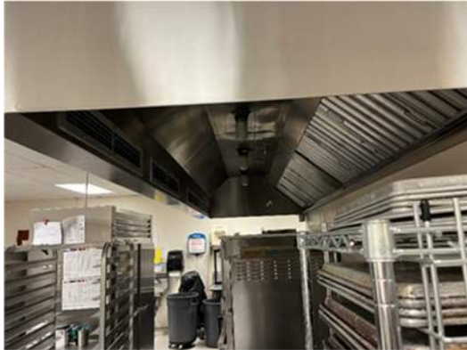
Existing grease hood
