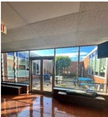
Courtyard at front entry
