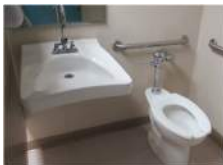
Existing Gang Toilet Plumbing Fixtures
