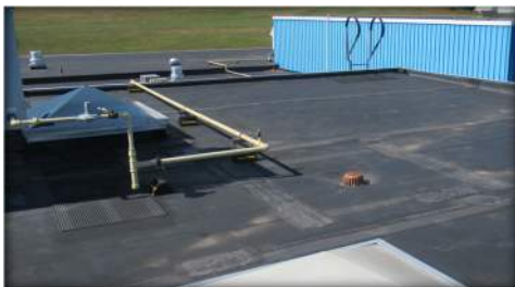
Existing Roof Drain
