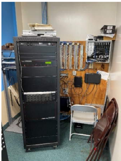
Existing Simplex 5100 public address head end
