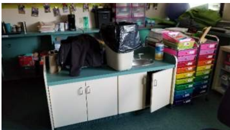
Typical classroom non-compliant sink
