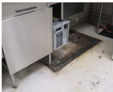
Existing Grease Trap
