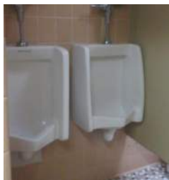
Existing Toilet Room Plumbing Fixtures
