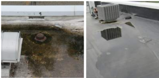
Existing Roof Drain
