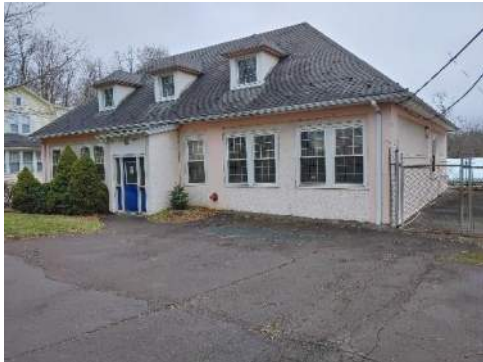
Abington Heights Maintenance/Facilities Building
