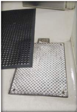
Existing Grease Trap
