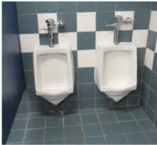
Existing Student Gang Toilet Plumbing Fixtures
