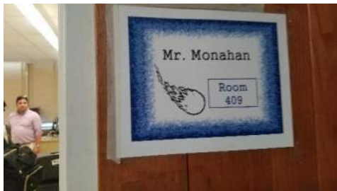
Non-compliant room signage
