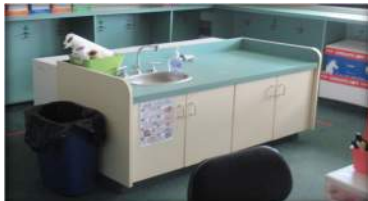
Existing Non-ADA Classroom Sinks
