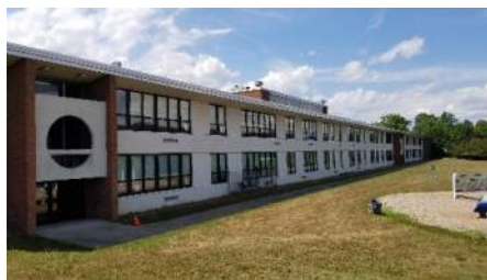
Rear façade with brick and concrete panels
