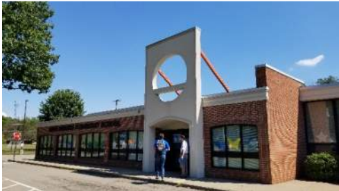
South Abington Elementary School Front Elevation
