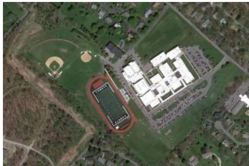
High School site
