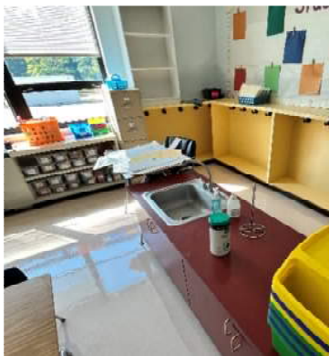
Typical sink in classroom
