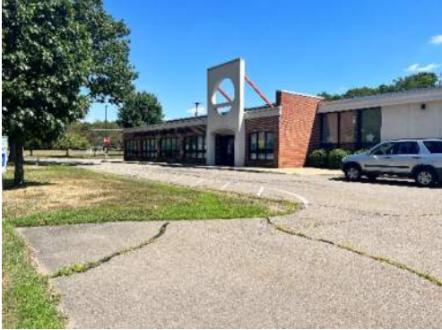
Cracking in parking area
