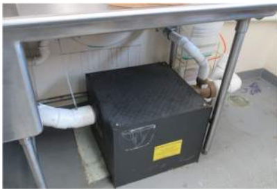
Existing Grease Trap
